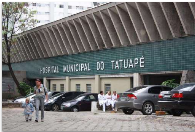
Fachada do Hospital HMCC
