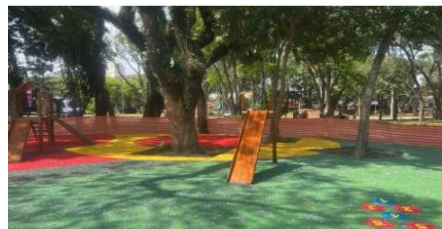
PISO EPDM E PLAYGROUND
