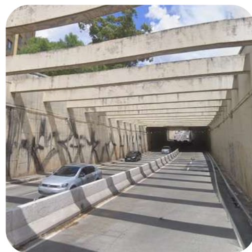
Túnel Takeharu Akagawa (a executar)
